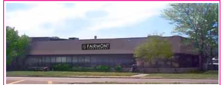
EASTERN UNITED STATES MANUFACTURING FACILITY
